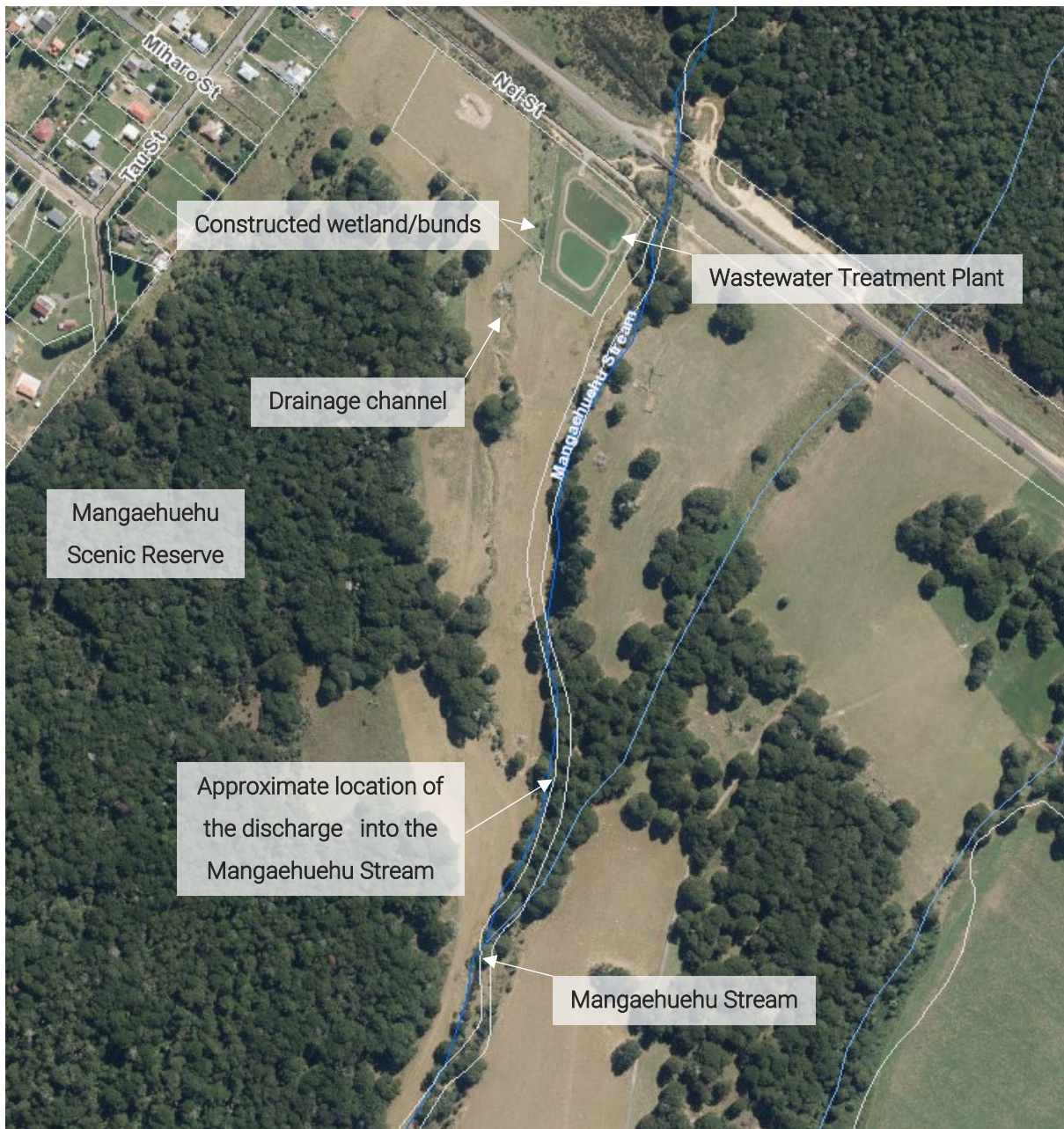
Figure 3 Discharge from the Rangataua WWTP into the Mangaehuehu Stream via a constructed wetland and drain
