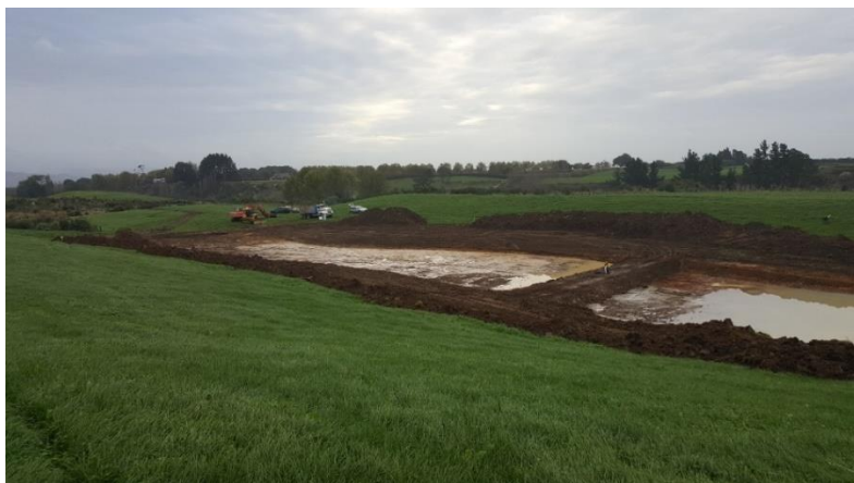
Figure 5: Wetland under construction with earth bund mid wetland. The bund overflow sill has been installed at 500mm above the base of the upstream wetland bay so that water depth never exceeds 500mm.
